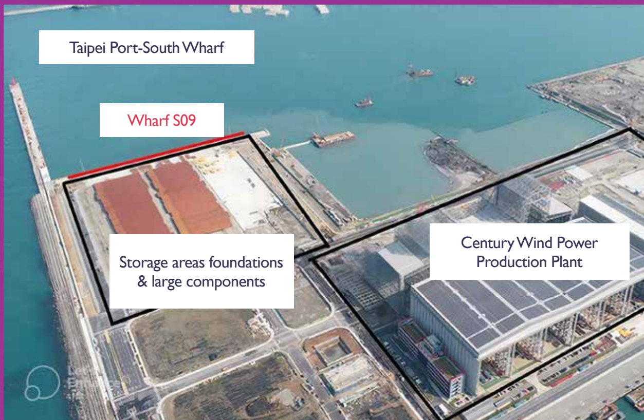
Figure 5 Taipei Port-Foundation Fabrication and Logistics Site
